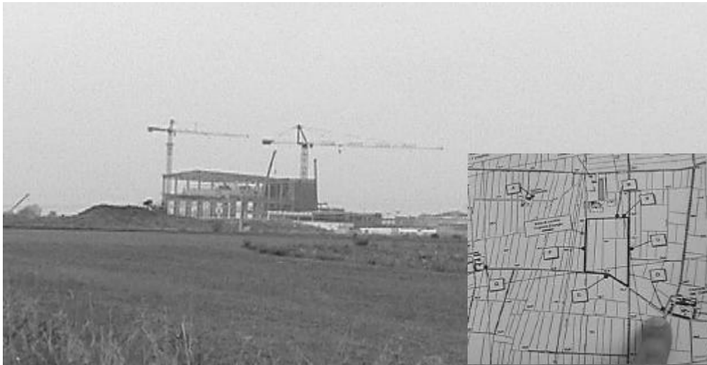
Figure 2: View of the Power Station under construction taken from one receptor
