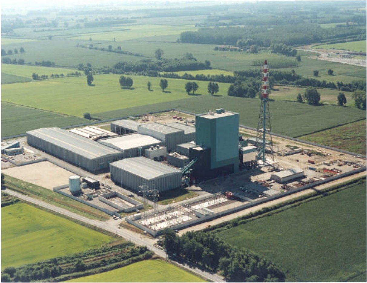
Fig.1 – View of the plant.
